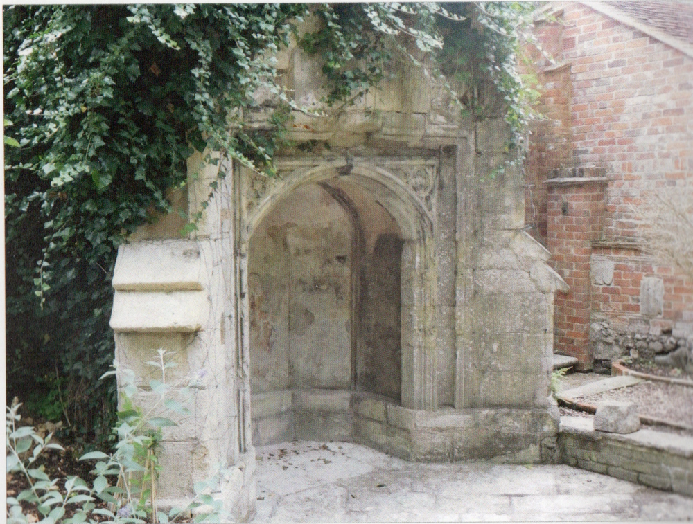
Transplanted doorway at 44 St Ann Street
